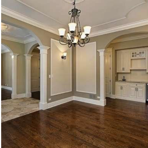
Figure I-5 Wall “picture” frame moulding
