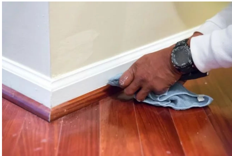
Figure I-4 Baseboard with shoe moulding
