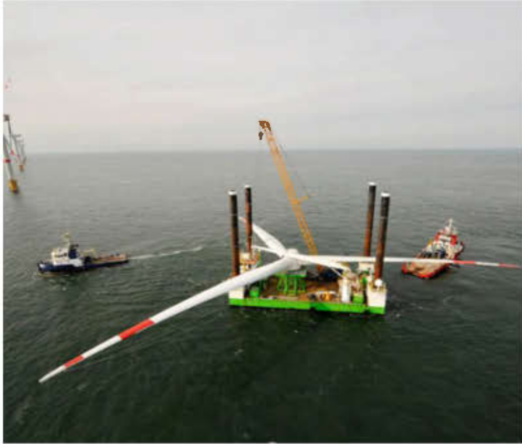
Transporting a rotor assembly loaded on a seajacking barge.
