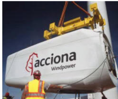
Raising the nacelle, containing the generator, for mounting onto the top-section flange.
