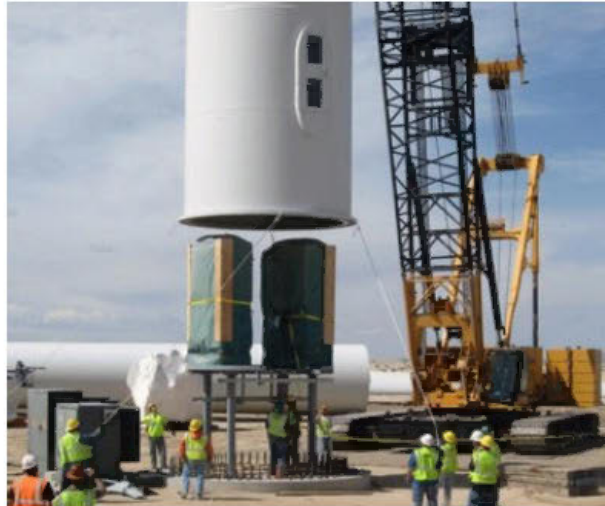
Lowering the base section onto the foundation platform and over the power unit.
