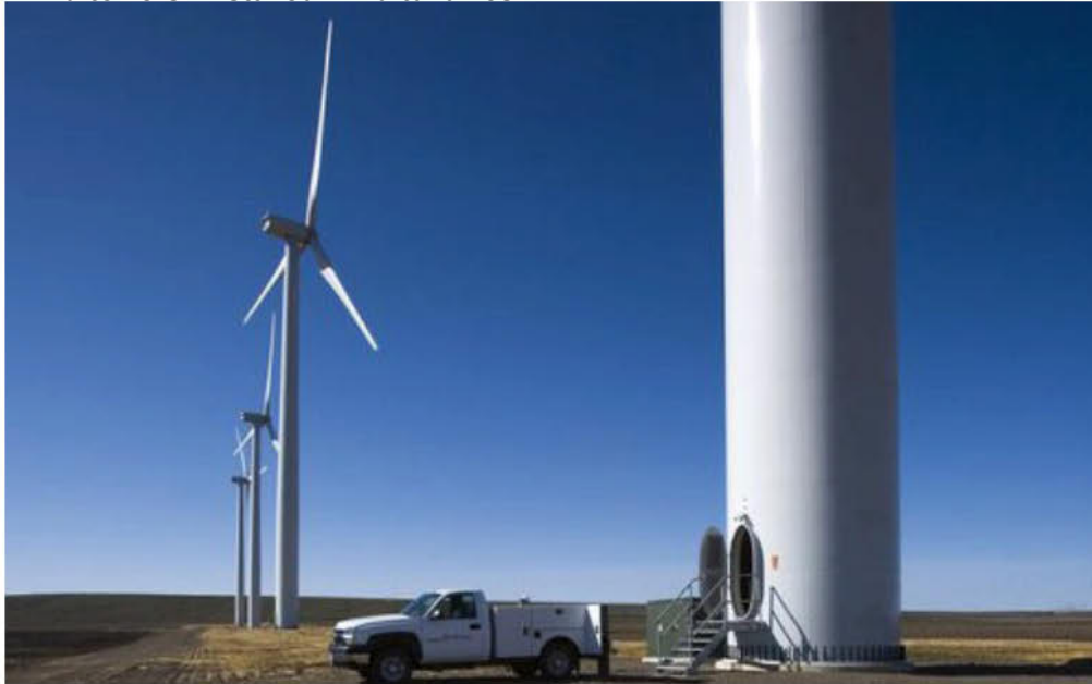
Figure I-3 Wind towers: Installed wind turbines
