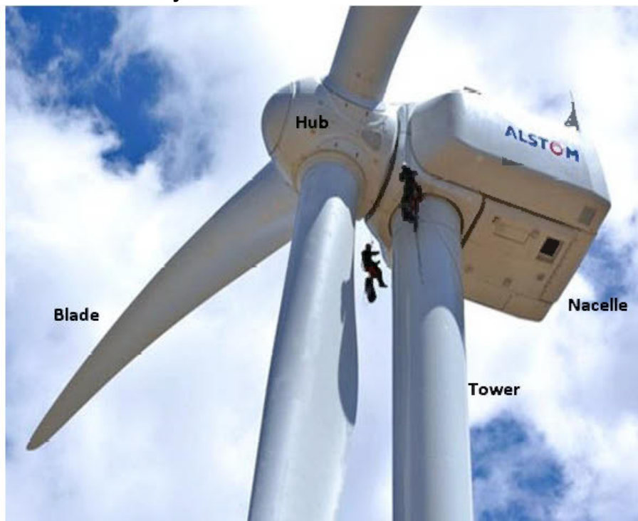
Figure I-1 Wind towers: Utility-scale wind turbine
