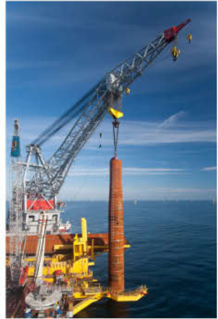
Hydraulic driving of the monopile.
