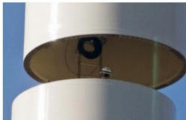
Positioning tower sections for bolting together the flanges.
