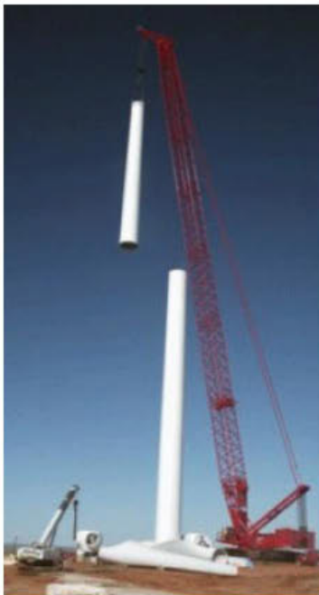
Raising and positioning the next tower section over those already in place.
