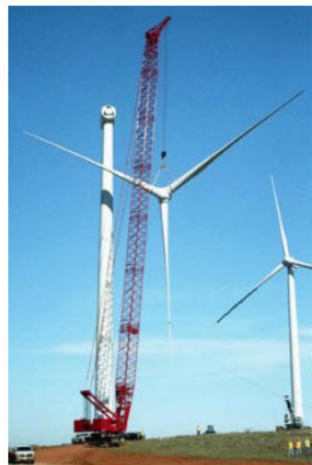
Raising the rotor assembly for mounting onto the generator shaft at the front of the nacelle.
