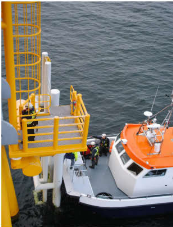
Transition piece with mooring fixture and ladders.
