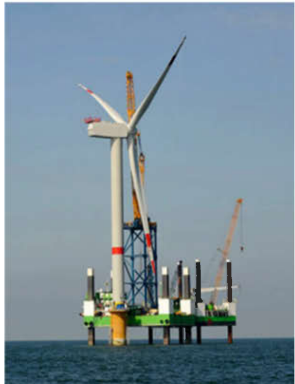
Installing the rotor assembly onto the nacelle.
