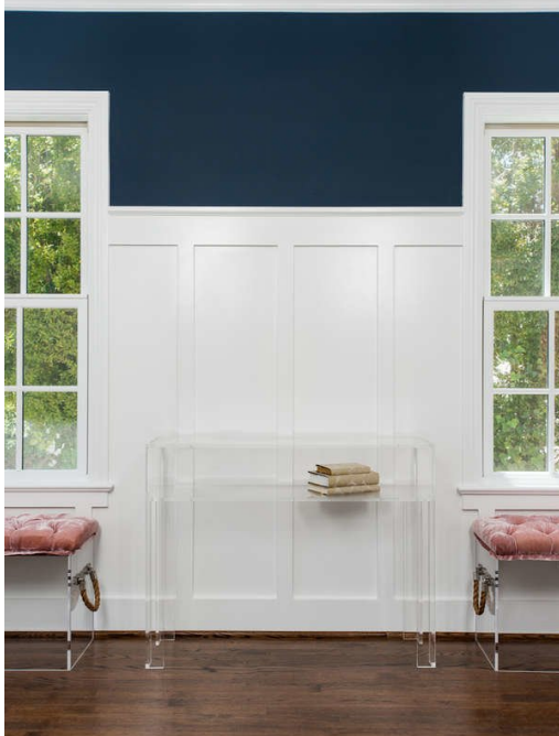
Figure I-7 Board-and-batten wall moulding
