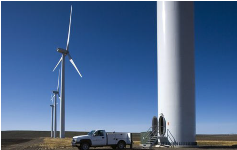
Figure I-3 Wind towers: Installed wind turbines
