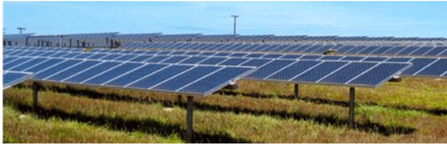
Figure I-6 LA Ola PV plant, a utility CSPV system on Lanai, Hawaii
