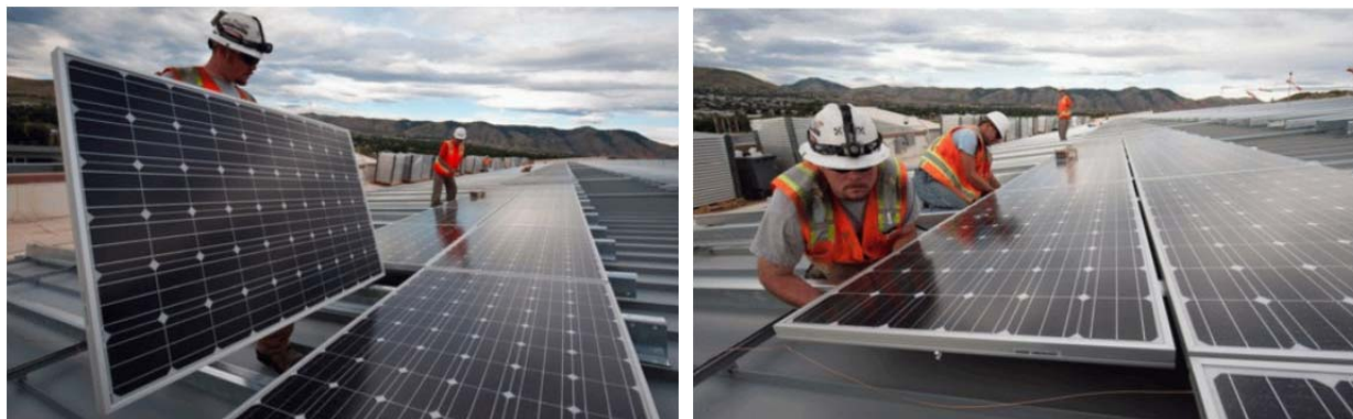
Figure I-5 Installation of a nonresidential CSPV system
