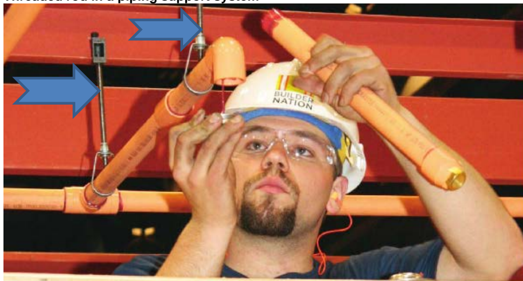
Figure I-1. Threaded rod in a piping support system
